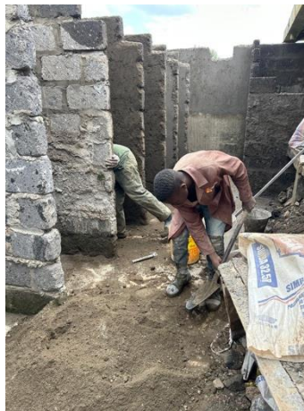
New toilet & shower blocks being built
